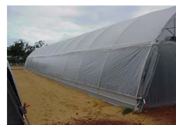
Roll up sides with winches
