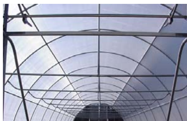
Fully braced frame
