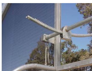
Rack and pinion vent drives
